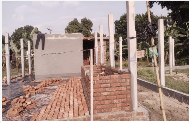
Farmers' Hub construction work in progress
